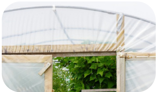
Armada Farm polytunnel
